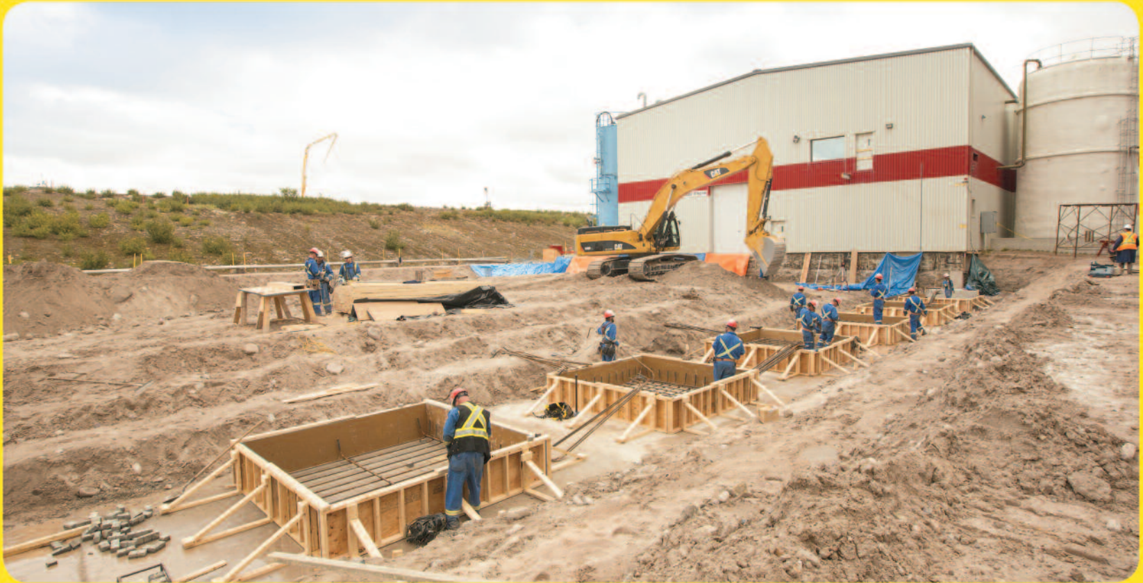
McClean Lake Mill Expansion, Northern Saskatchewan
